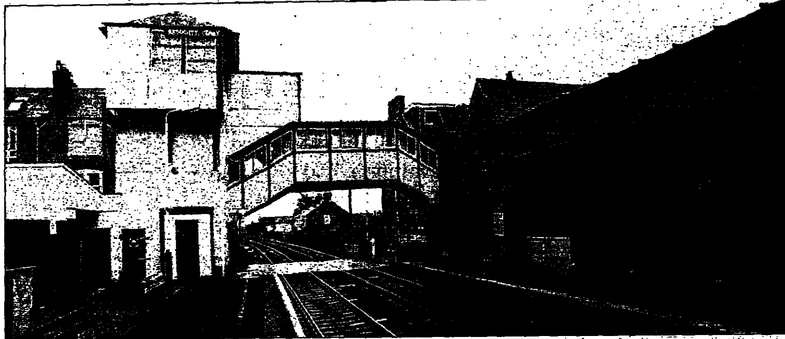
Broughty Ferry station, near Dundee, opened in 1838, a year after the London to Birmingham railway. The footbridge was added in 1886
